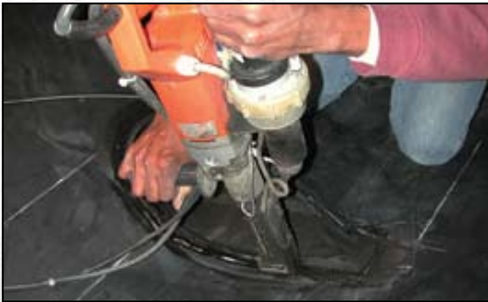
A hot air welded joint provides zero leakage.
