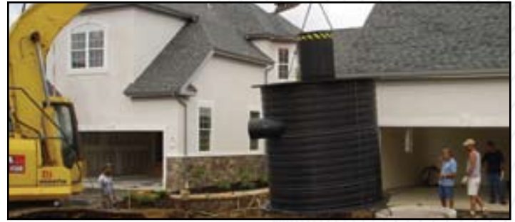
Aqua-Swirl ® installation at a residential development in PA.
