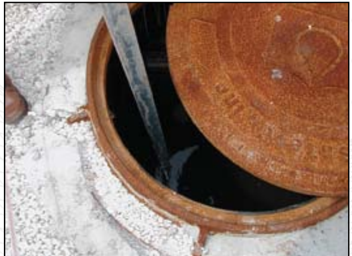
Inspection of an AquaShield™ stormwater treatment system.
