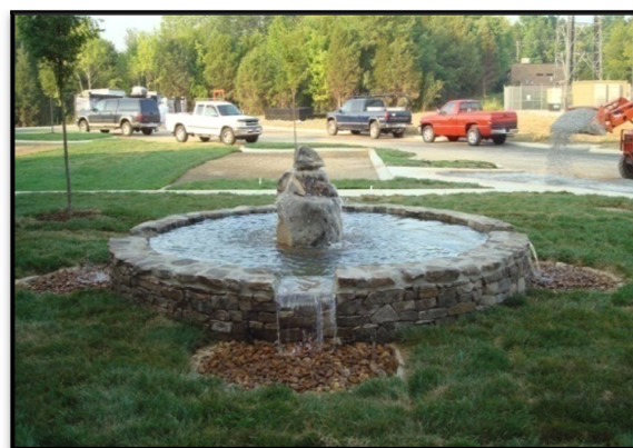
Figure 2. Water fountain uses water harvested from stormwater and roof runoff. The fountain sets directly above the underground modular storage unit.
