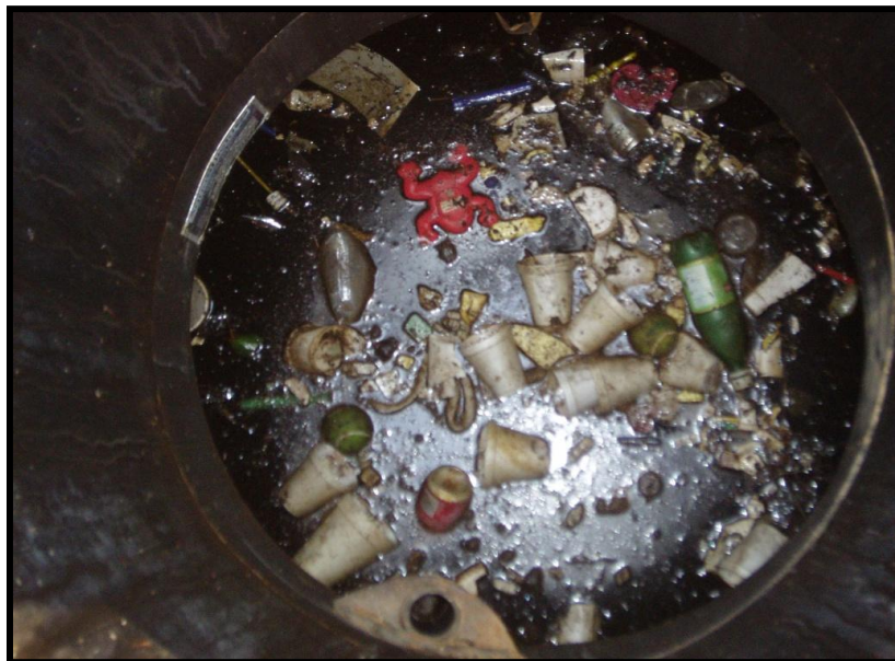
Figure 3. Trash and floatables in an AS-6. Vent pipe is visible in the bottom of the photograph.
