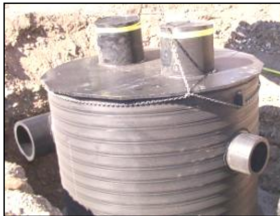
Pretreatment HDS chamber component of the Aqua-Filter™ System. Note tangential inlet and outlet piping.
