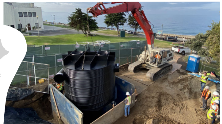
The 12,400 lbs, 12-ft AS-12s being installed
