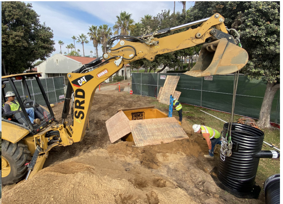
The Aqua-Swirl® AS-2s dry weather unit being installed
