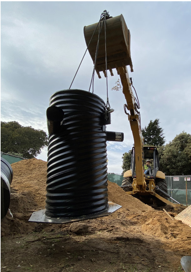
The Aqua-Swirl® AS-2s dry weather unit being installed
