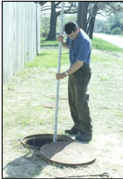
Sediment inspection using a stadia rod
